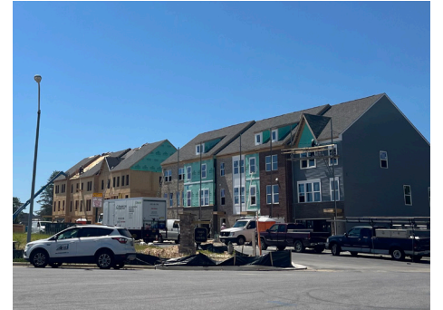
Construction has begun on the Oaks at Laurel.
